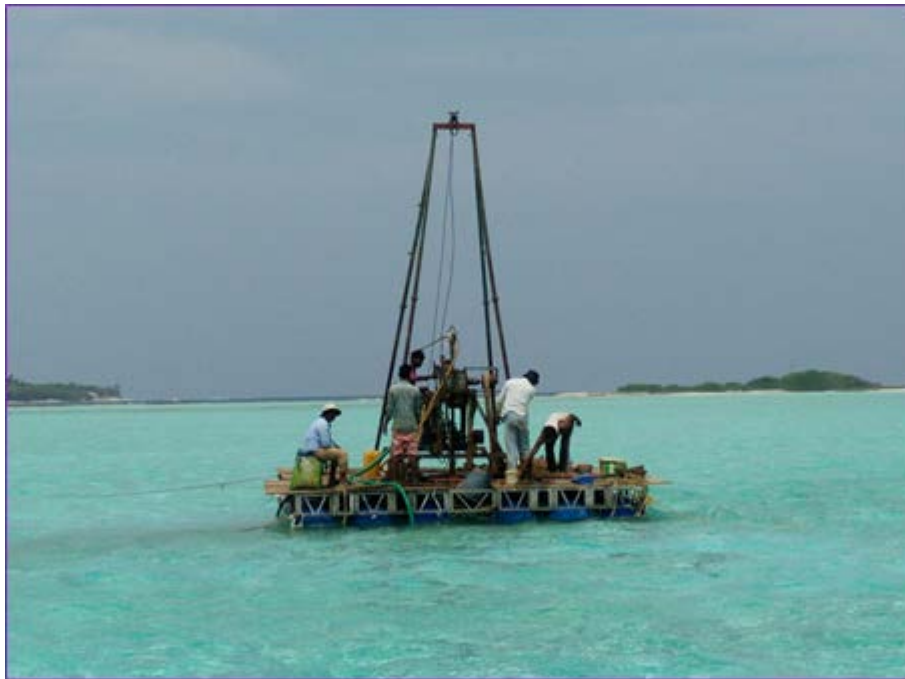
Figure 2.2: Image showing borehole drilling plat form and equipment
