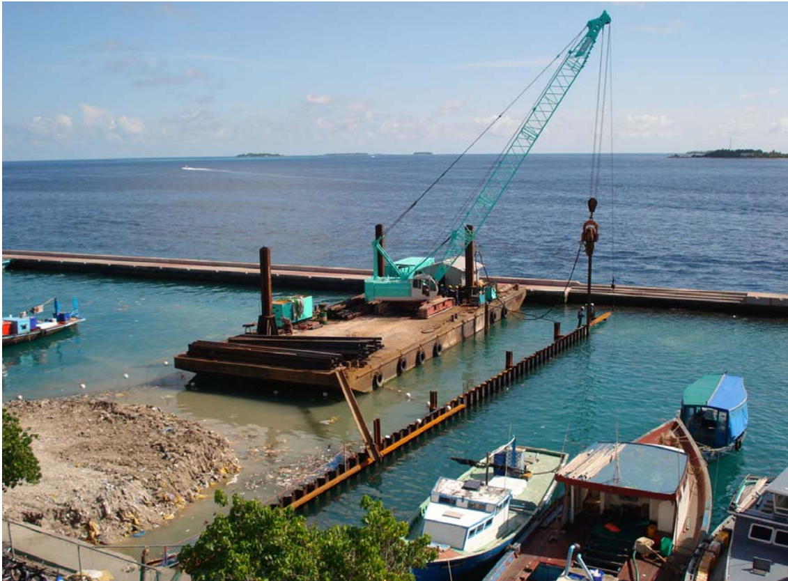
Figure 6: Barge used for sheet piling for the proposed New Fish Market.
