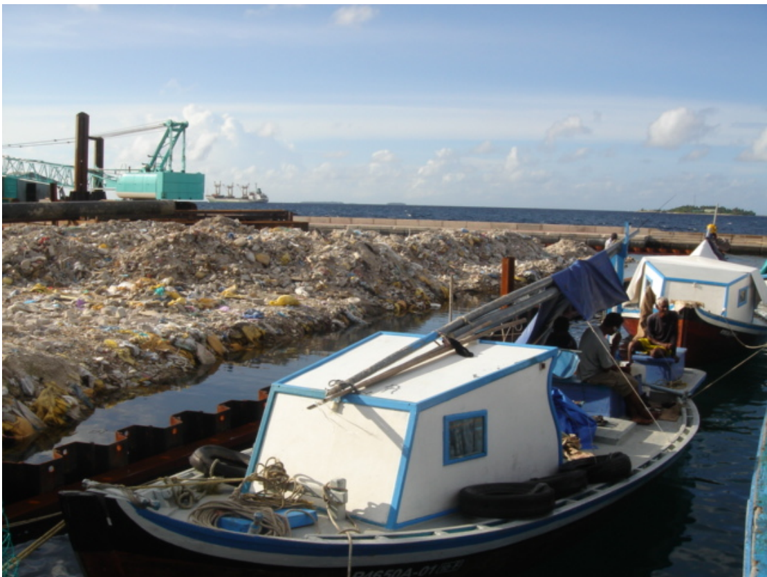
Figure 3: Part of reclaimed area for the proposed new fish market.
