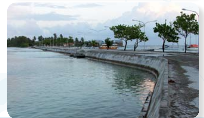
Causeways were constructed during WWII by the British military to facilitate the movement of troops and equipment between the islands. These causeways have led to a change in the circulation patterns of water flows in and out of the lagoon. Photo: Melanie King.
