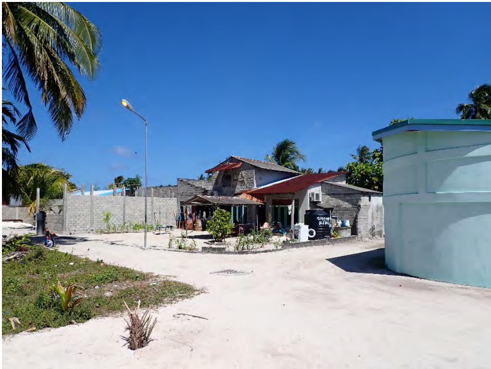
Figure 11. Construction site adjacent to IWRMC site
