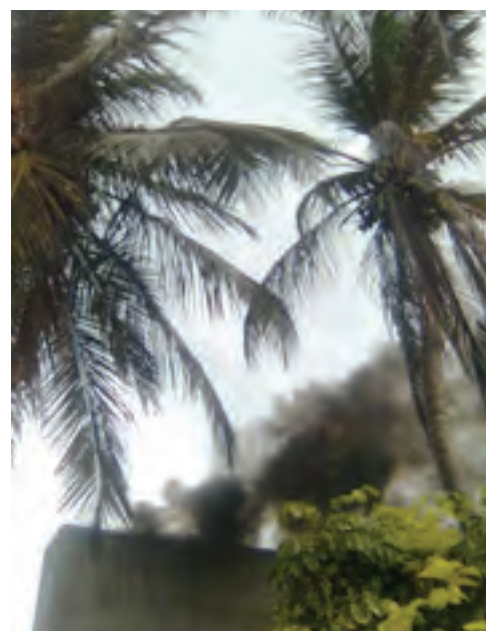
Black smoke emitted from a small powerhouse
