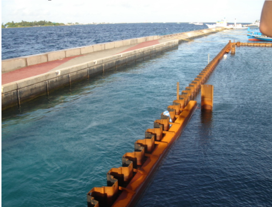
Figure 9a: Shows channel for water movement.
