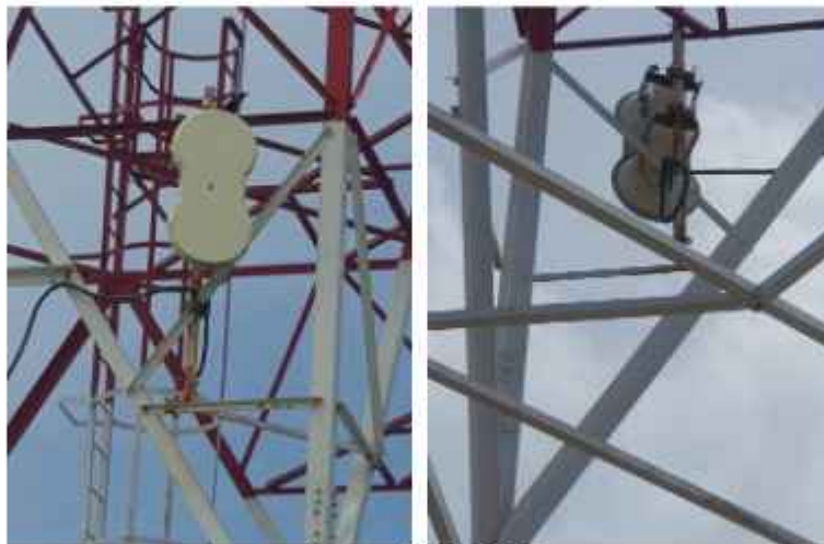
Figure 17: Current status of the Malé radar air fiber data link to MMS head office
