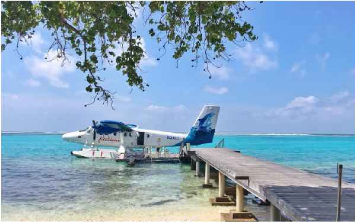
Figure 3: Seaplane pier in the south of the Addu International airport
