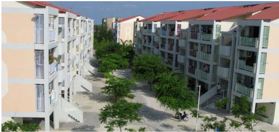
Apartment blocks in Hulhumalé'
