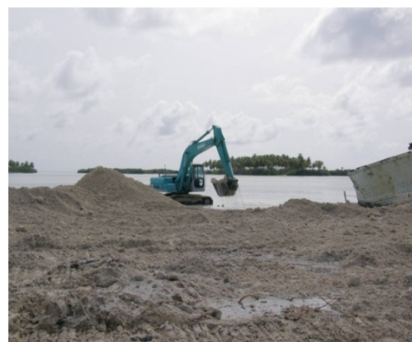
High cost of material forces the public to use coral and sand from the beaches for construction
