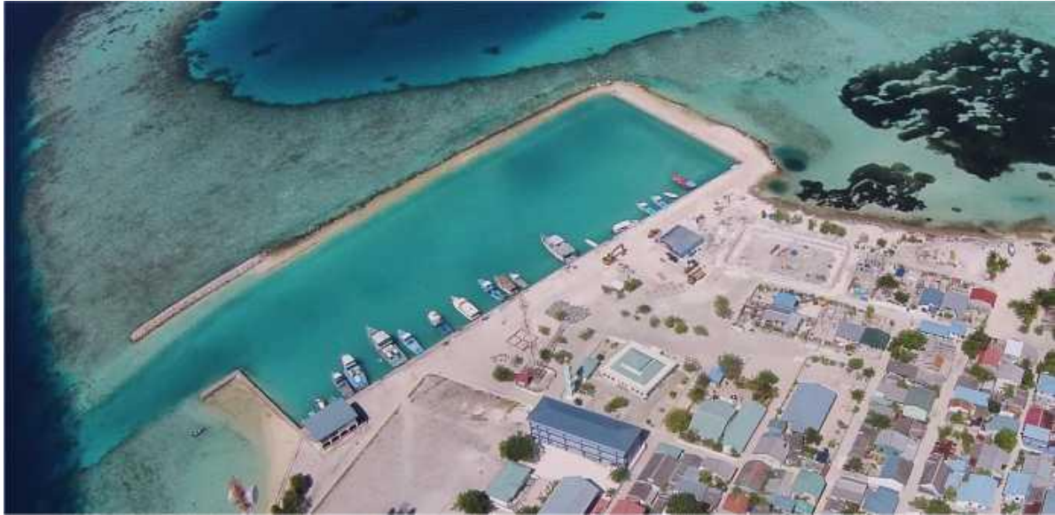
Figure 19: ongoing harbour development project
