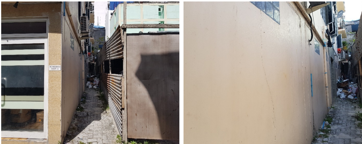
Figure 18: Building to the west of the project site
