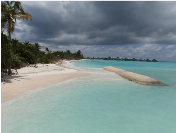
Geotube with accumulated sand (Englund, 2014).
