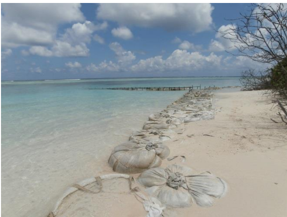
Seawall made by jumbo sandbags protecting the beach (Englund, 2014)
