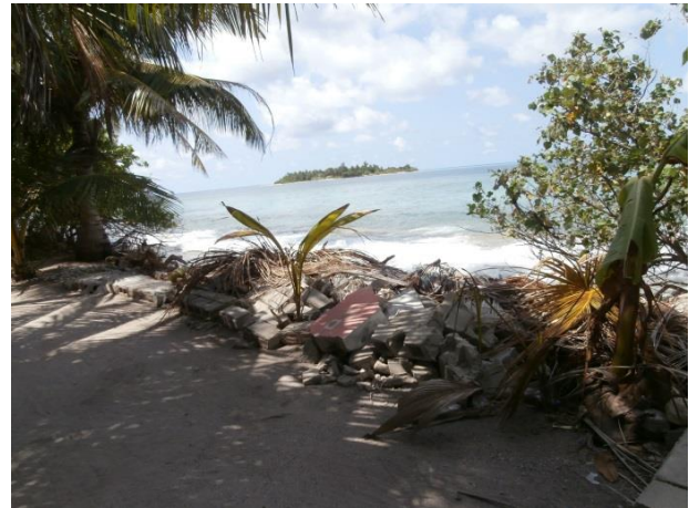
A wall of building material, stones and garbage to protect from erosion (Englund, 2014).
