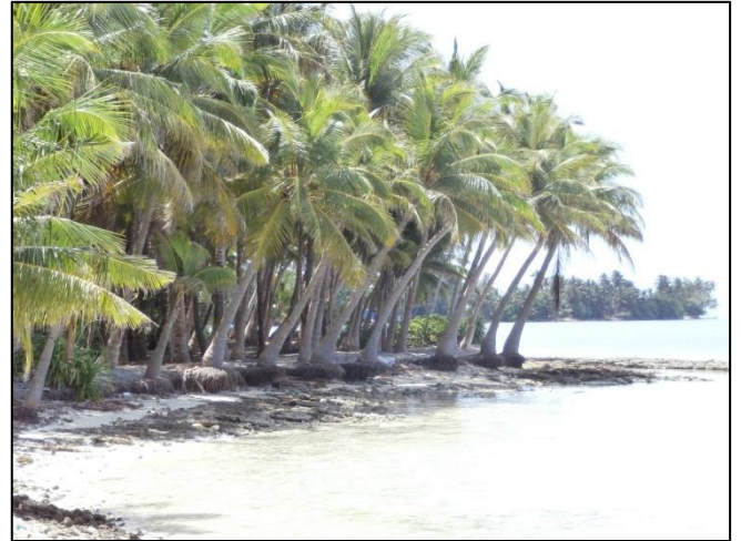
Erosion on the western part of Maavah.
