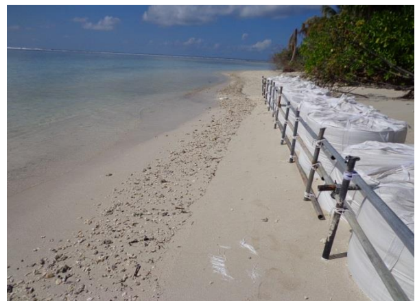
Seawall made by jumbo sandbags protection the beach (Six Senses Laamu, 2014).
