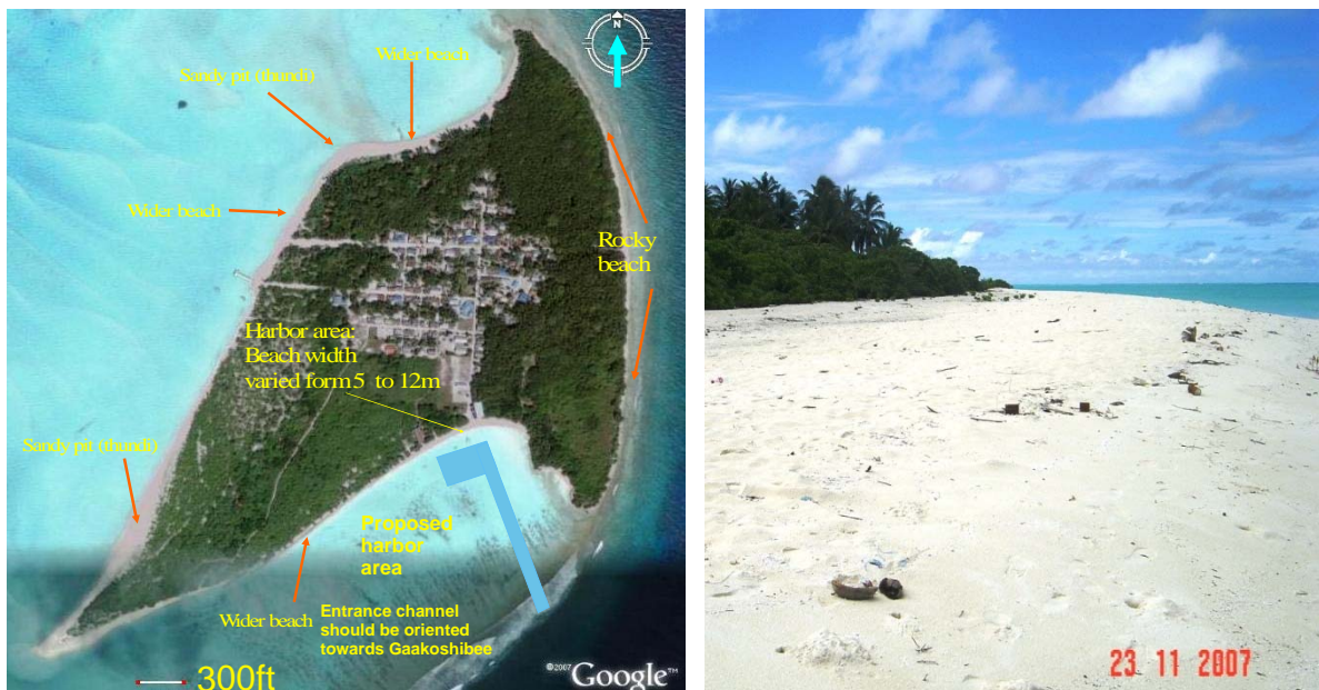
Figure 8: Beach widths of Bilehahi (left). Wider beach was found at the northern side of harbor (right)
