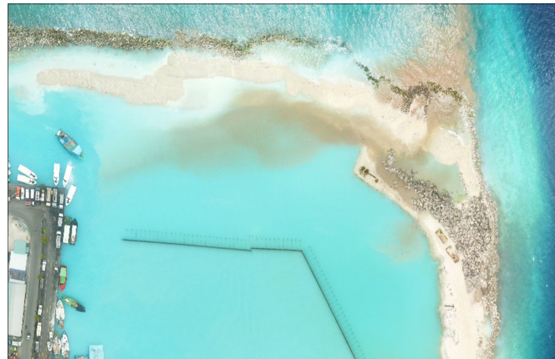
Tetrapod breakwater moved and sand bund created at the southwest end.
