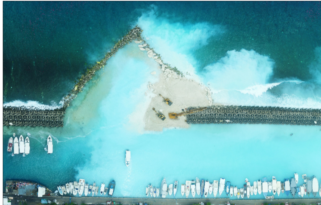
New channel into South Harbour being dredged. The sediment moves slightly westerly as per wind-induced currents at the time (early May 2016)
