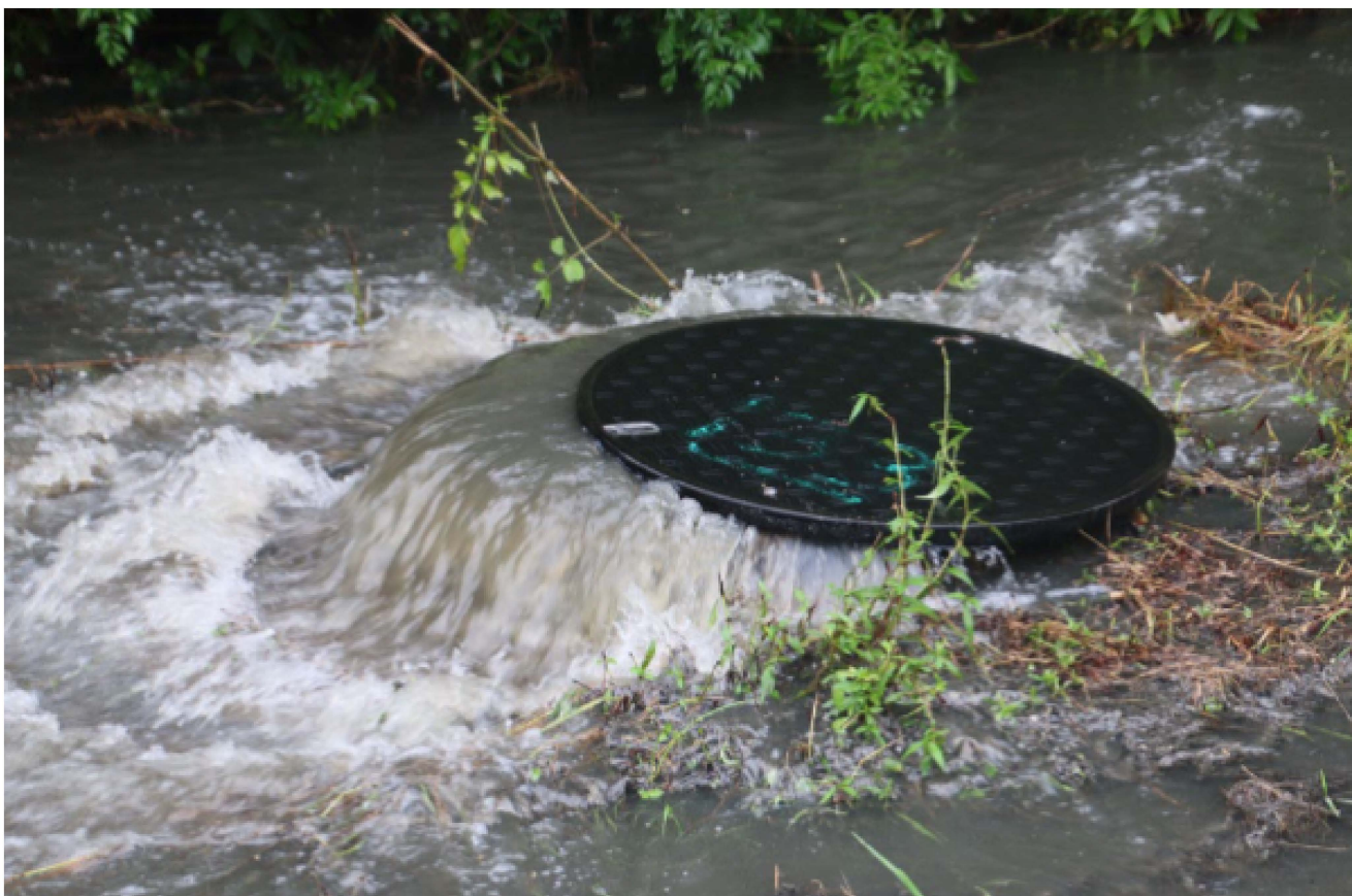
Figure 11: Sewerage overflow from a sewer manhole (Source: Ministry of Environment, 2021; Photo: https://www.apr.org/news/2019-06-06/alabama-probes-fish-kill-after-sewage-spilled-near-creek )
