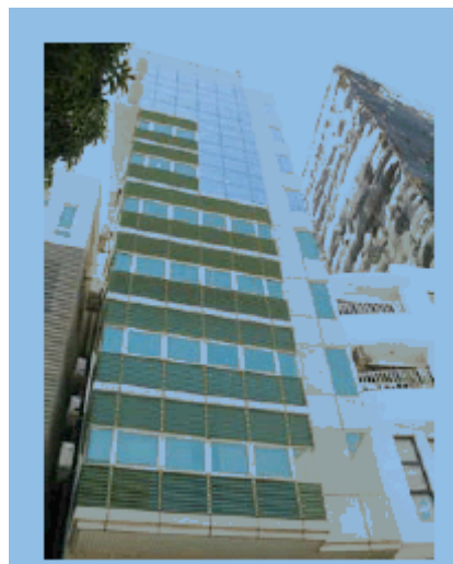
Fig 7. ADK tower 12-30m west of the site.
