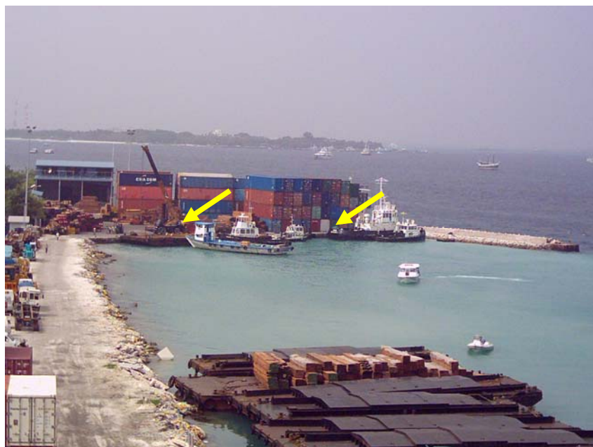
Figure 4: Temporary loading and unloading area for construction phase.
