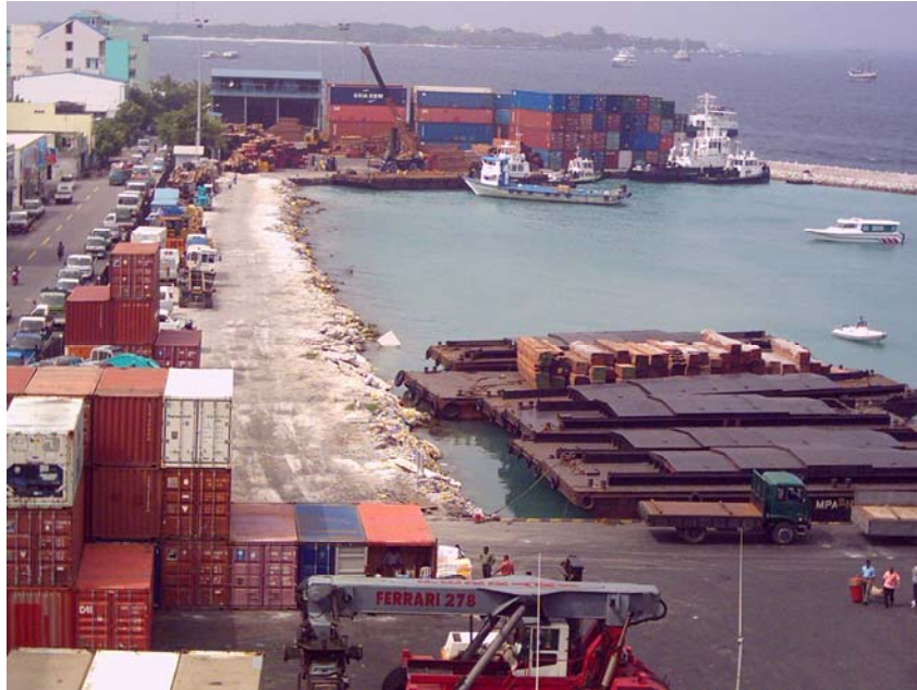
Figure 12: About 20m wide area which had been reclaimed previously
