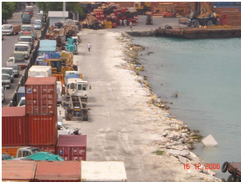
Figure 11: West side of project site is paved area. This area is used for storing cargo containers and woods
