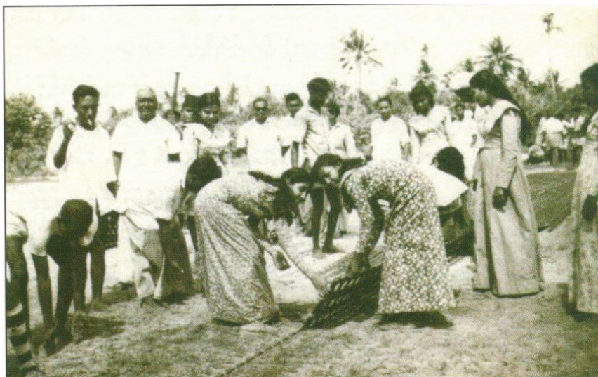
Figure 5: Volunteers dismantling Martson Mat at Hulhulé Airport
